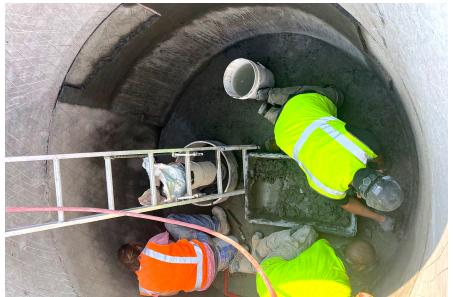
Blackwater Engineers were satisfied with the concrete's long-term protection that included a combination of Admix C-500, Megamix II with Bio-San and Bio-San C500.
